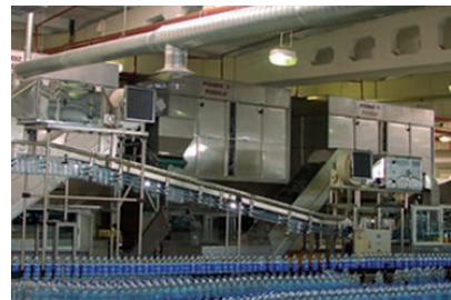
Unscrambler, Silos and Air Conveyor installation
