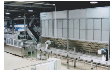
Unscrambler, Silo and Air Conveyor installation
